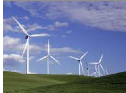
Wind turbines (iStockphoto)
